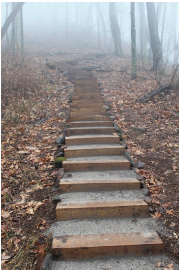
White oak steps leading out of the parking area on the Ridge Trail. (Z. McGee)
