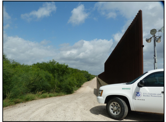
Looking down the border wall at the Lower Rio Grande NWR. Note the wide swath of cleared land, the cement wall, the 30-foot fence, and the lights. (Photos by Nancy Sorrells)
