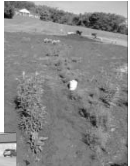
BEFORE & AFTER —The DCR water quality project retrofitted a poorly functioning and ugly stormwater management basin (left) into a rain garden (above) planted entirely with native plants. The plants provide a nicely landscaped garden area and clean the rainwater before it heads to the South River (a tributary of the Shenandoah River). (Photos by Nancy Sorrells)
