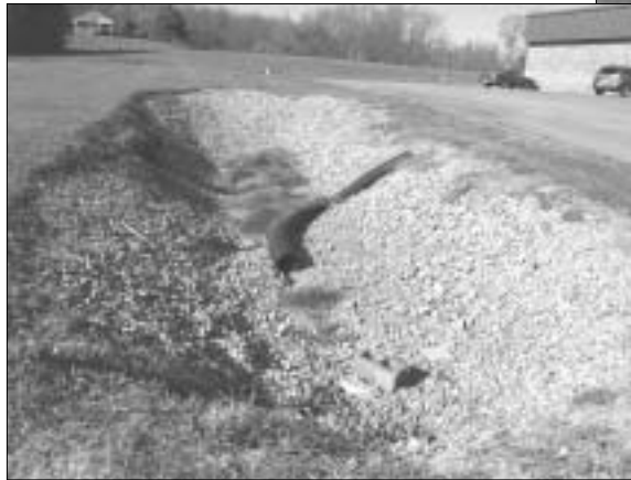
BEFORE & AFTER —The DCR water quality project retrofitted a poorly functioning and ugly stormwater management basin (left) into a rain garden (above) planted entirely with native plants. The plants provide a nicely landscaped garden area and clean the rainwater before it heads to the South River (a tributary of the Shenandoah River). (Photos by Nancy Sorrells)
